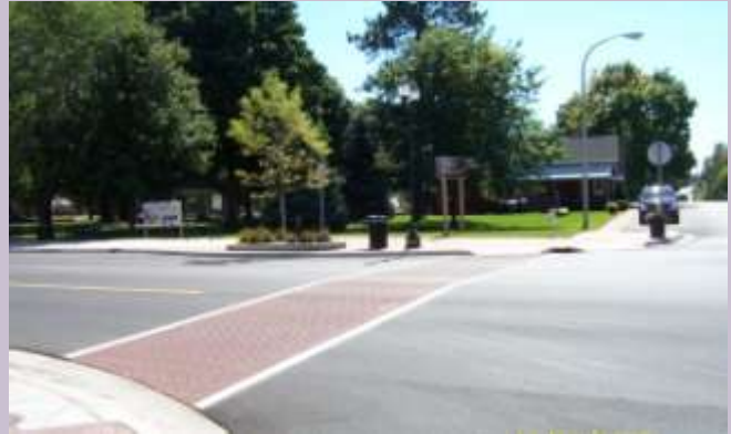
Example of how driveway design can draw attention to pedestrians in the crosswalk using color and texture within the pavement surfaces.
