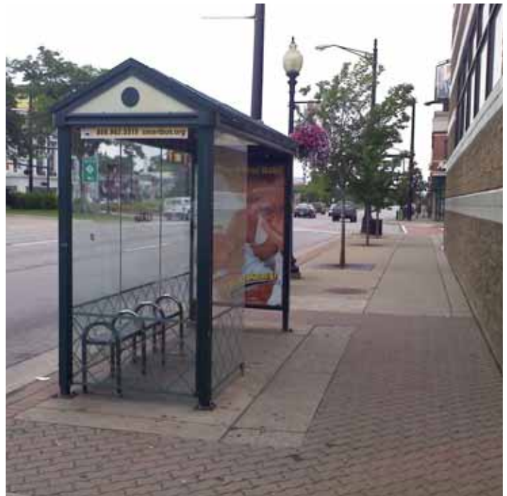
A new SMART bus shelter in Frensdale, MI. The bench and roof at this shelter help protect bus riders from the elements while waiting for a bus.
